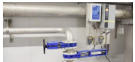
AVK knife gate valves with linear actuators on a reject water pipeline. The linear actuators were chosen, since they are energy efficient compared to actuators using compressed air
