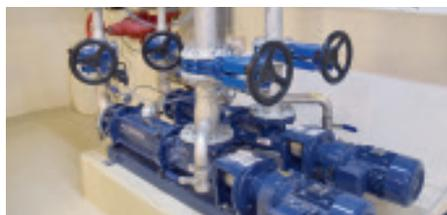
Sludge from the bottom of the clarification zone in the DEMON® tank is pumped back to the process as return sludge, and excess sludge is pumped into a cyclone, where anammox bacteria are sifted out.
