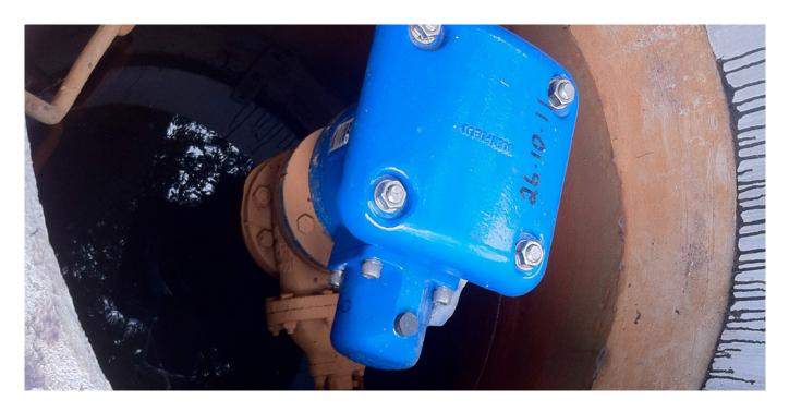
AVK's Large Orifice Series 851 Air Release Valves incorporate the exclusive Glenfield Aerokinetic Principle which prevents premature closure while air is being released from a pipeline.
